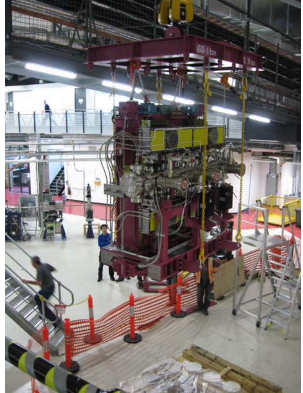
The 2metre undulator was lifted over the ring wall into the internal area of the storage ring in preparation for installation inside the storage ring in October.
