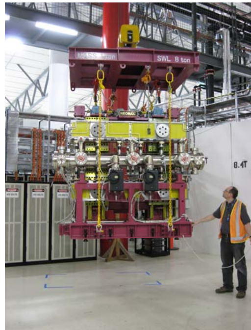
The 2metre undulator was lifted over the ring wall into the internal area of the storage ring in preparation for installation inside the storage ring in October.
