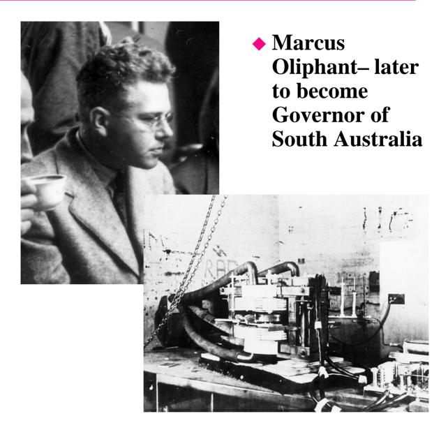
The Arsenal Synchrotron- Late in World War II the Woolwich Arsenal Research Laboratory in the UK had bought a betatron to "X-ray" unexploded bombs in the streets of London. <u>Frank</u> Goward converted the betatron into the <u>first "proof</u> <u>of principal"</u>
