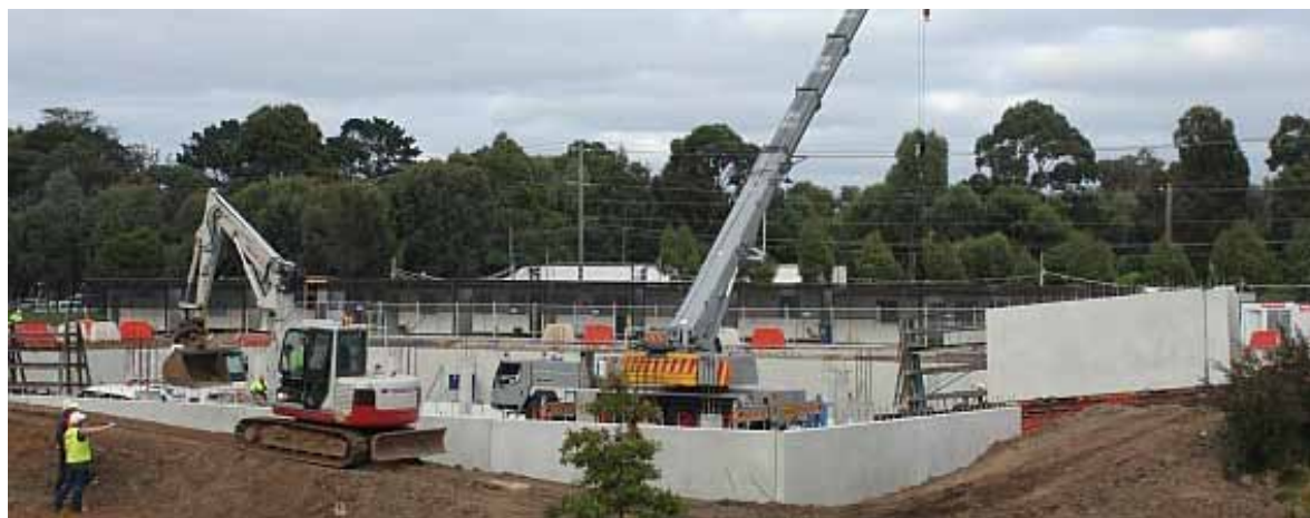
(17 March 2011): construction work for NCSS building.
