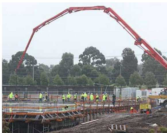
(14 April 2011): pouring concrete in the rain for the NCSS building.
