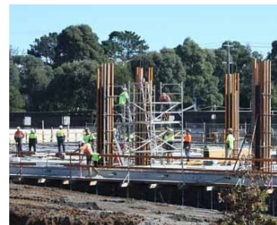
(21 April 2011): progress with construction work for NCSS building.
