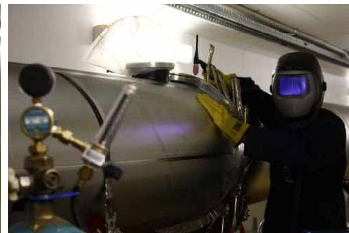
Above left: construction of the vacuum transfer line in the IMBL tunnel
